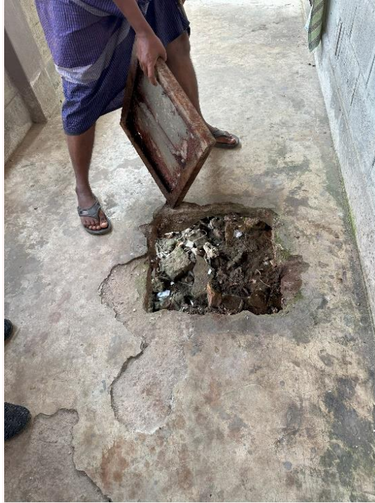
Lack of adequate weatherproofing (driving rain)
