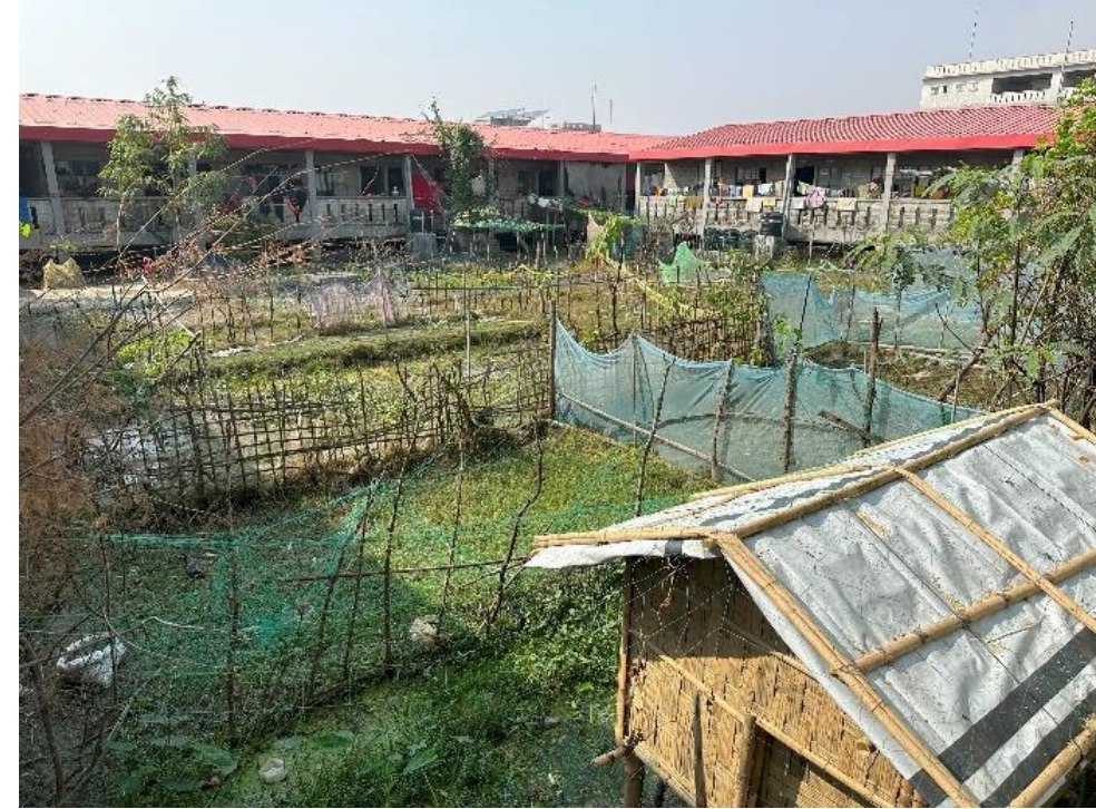
Problems of central courtyard
